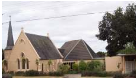
View from South Valley Road after 1990 extensions
